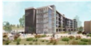
Mesa Court Housing Expansion
